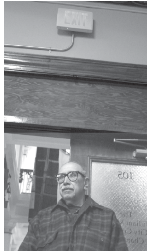
Eddie Costa showing the exit sign and emergency lights recently installed in the City Council Chambers.
