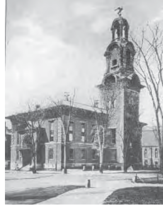
City Hall before the 1923 expansion City Hall was erected in 1849
