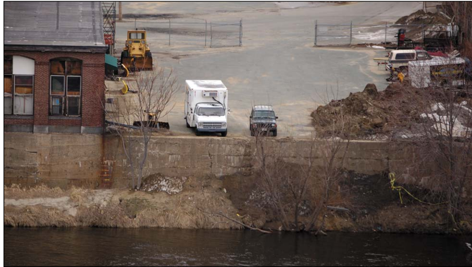
This picture was taken 03/27/07, seven days after the storm, from the opposite side of the river, that shows a dark spot by the retaining wall, that could be silt been pushed from the lot, over the retaining wall.
