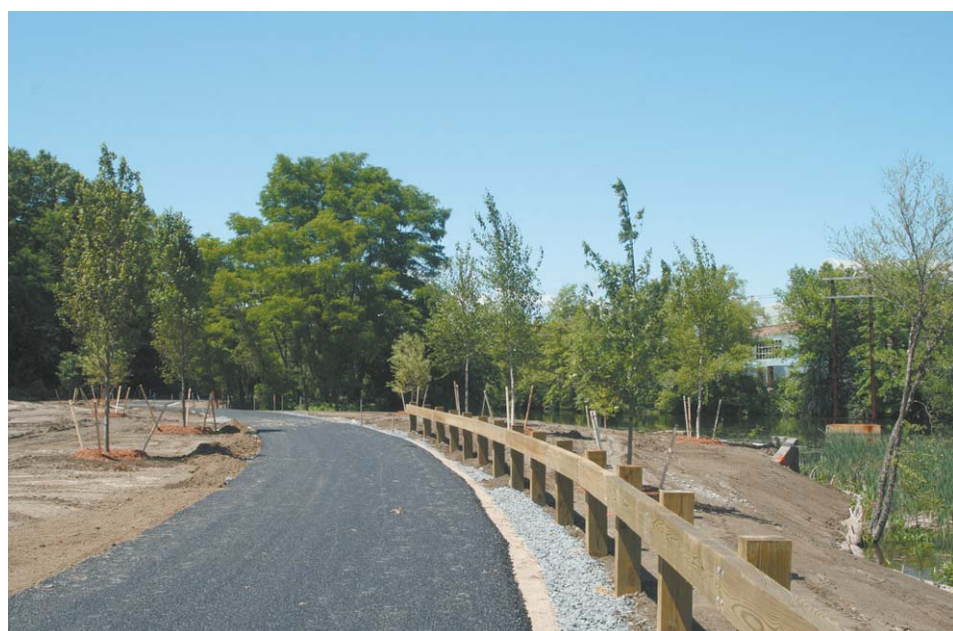
Another view of the park under construction.
