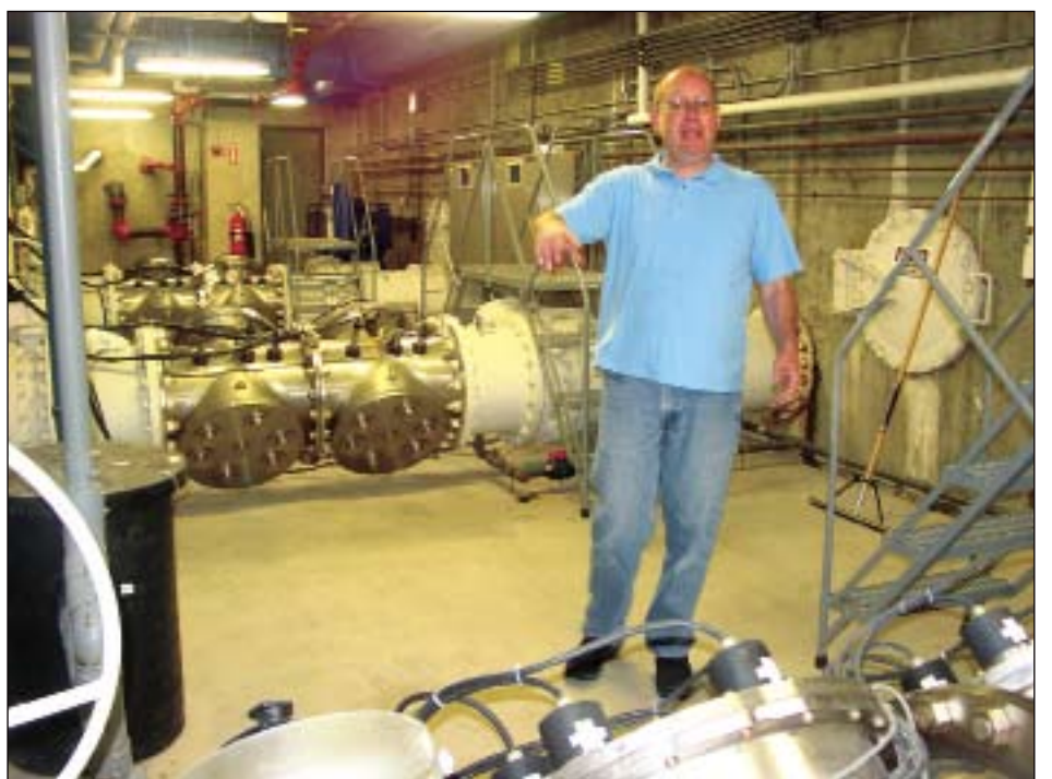
Lawrence has six ultra violet turbines. Four are used all the time and the others are a back-up.
