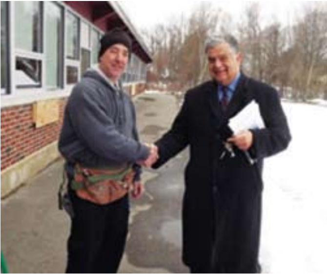
(L-R) Window installer and Mayor James J. Fiorentini at the Whittier School.
